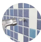
02. Fix the plastic tube into the hole
